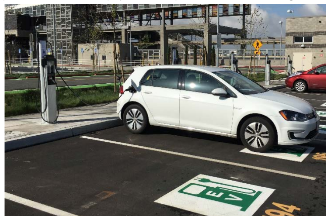
EV Charging Station at the Warm Springs, CA BART Station
